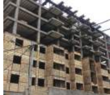
63-unit project on Luqman Street
