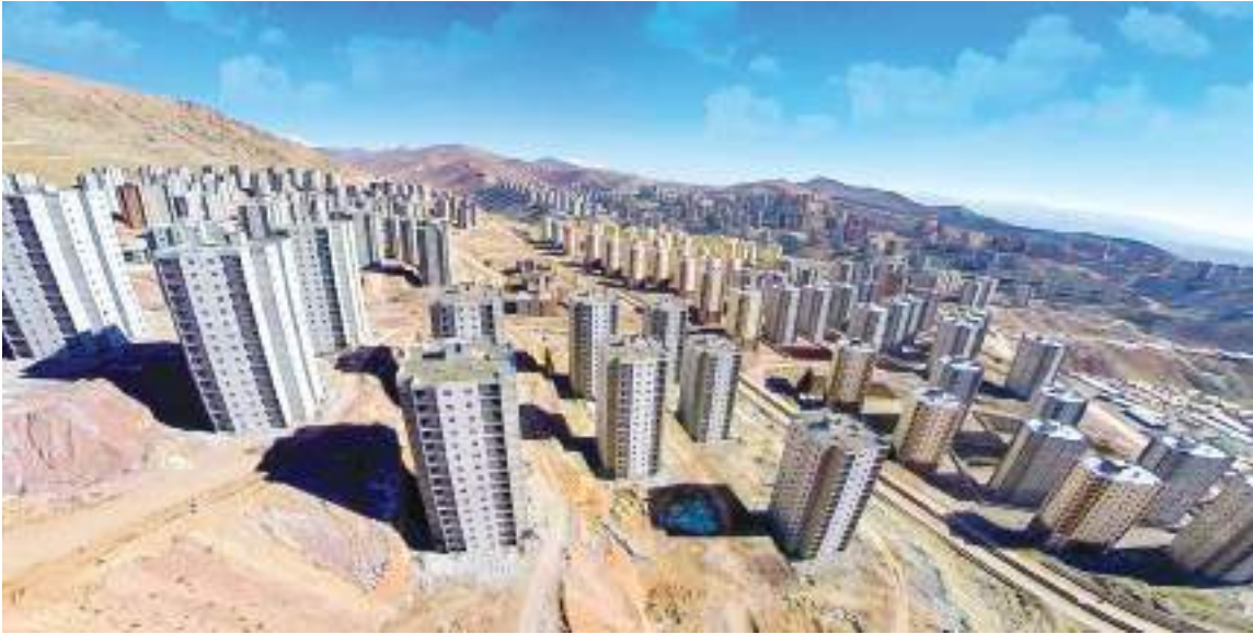
Kozo 35,000-unit project
